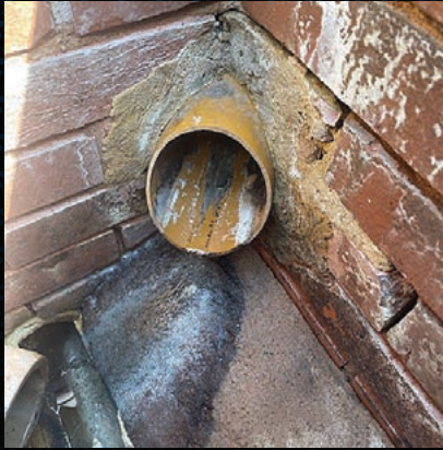
This chamber wall looks great from above... ...but not so good from below the service pipe.
