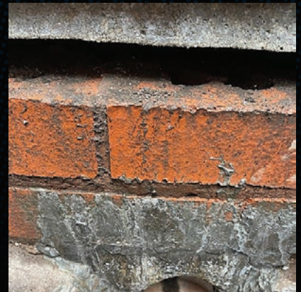
The underside of the frame can reveal large rodent entry points.
