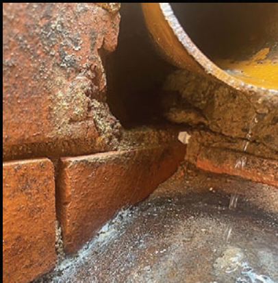
This chamber wall looks great from above... ...but not so good from below the service pipe.
