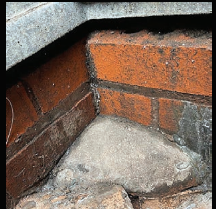
The underside of the frame can reveal large rodent entry points.
